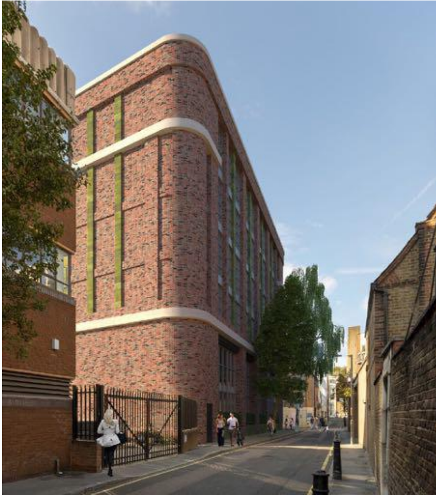
View looking west on Copperfield Street
